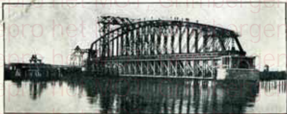
A span of 372 yds in length. (Double line Railway Bridge over the Meuse at Heusden (Holland).
